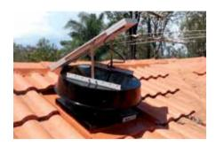
roof space temperatures to be brought down relatively close ambient. Controlling the roof-space temperature will reduce the temperature in the house - and if you have ducted air-conditioning reduce running time - whilst also increasing efficiency - saving you hundreds of dollars every year.
