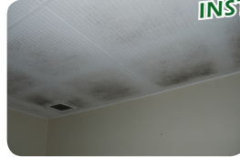
Mould on ceiling as a result of poor ventilation.
