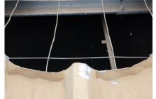
8. Fold up the lip on the lower side of the hole. This provides an extra physical barrier to prevent leakage
