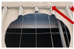
6. Remove the 5 bolts on the roof. If these are not removed then the flashing will not sit flush to the roof and will leak.
