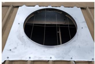
10. Place flashing base and hold in place by using a tech/roofing screw. Trick – Use the outside of the tin snips to secure a snug fit between the flashing and the roof.
