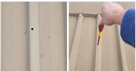
2. To check the positioning of the unit and avoid obstructions in the roof space, drill a small hole in the centre of the outlined flashing hole (pictured). Drop a screwdriver into the hole and have someone inside let you know if it is in a good position.
