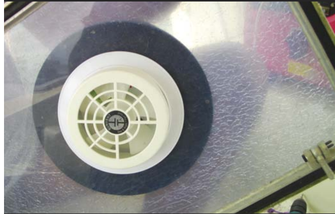
Insert the vent and put inner seal in place.
