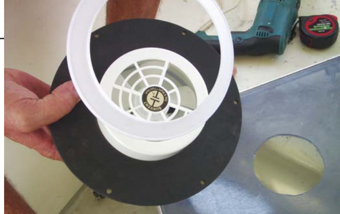
Remove masking tape and prepare vent to go into the hole
